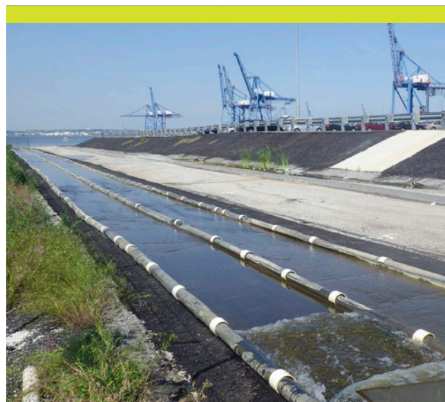
Located at the Port of Baltimore's Dundalk Marine Terminal, this algal turf scrubber takes up nutrients from the water, thus minimizing the major cause of water pollution in the Chesapeake Bay region.
