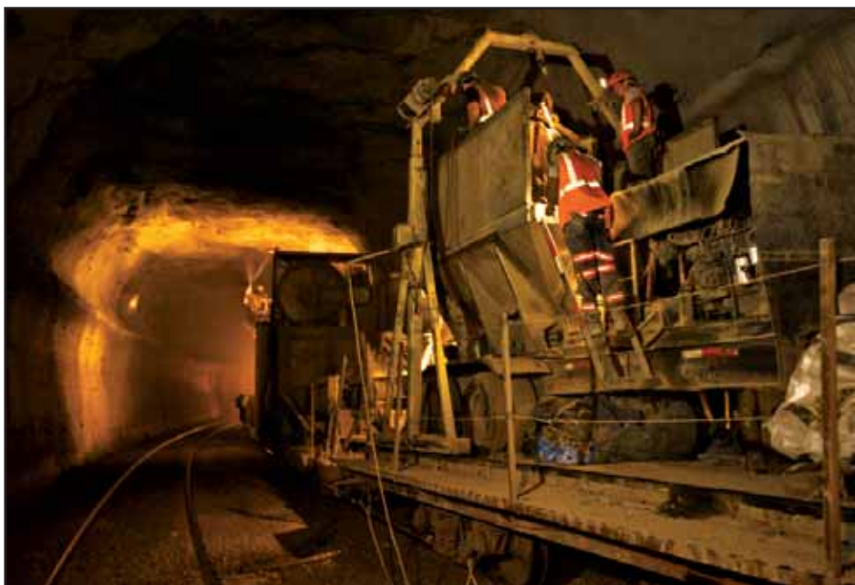
The Heartland Corridor improvements raised clearances in 28 tunnels on Norfolk Southern's line, allowing passage of double-stack trains.
