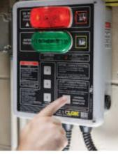
Rotating-hook restraints feature a hook that locks to the trailer's rear impact guard. A lighted control panel communicates the trailer's locked status to forklift operators and truck drivers.
