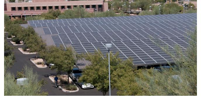
Avnet flipped the switch on a 1,000-kilowatt, 3,724-panel solar project that provides approximately 60 to 65 percent of the energy for its headquarters in Tempe, Ariz.
