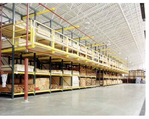
**LIGHTEN UP.** Diffusing skylights in this home improvement center warehouse in Silverthorne, Colo., increase daylight and reduce electric lighting and cooling loads.
