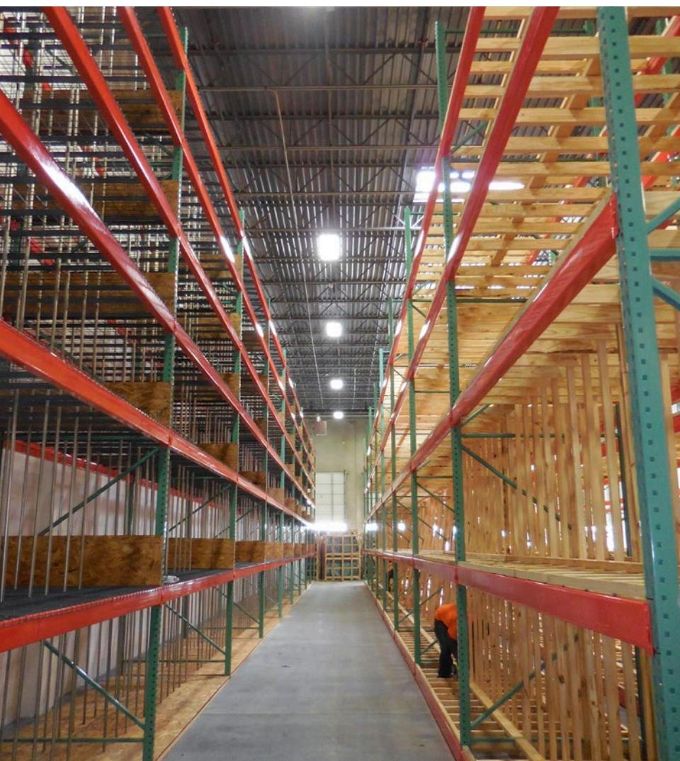
**Pushback racks can increase storage capacity in a distribution center by about 50 percent by stacking pallet positions up to six deep from front to back.**
