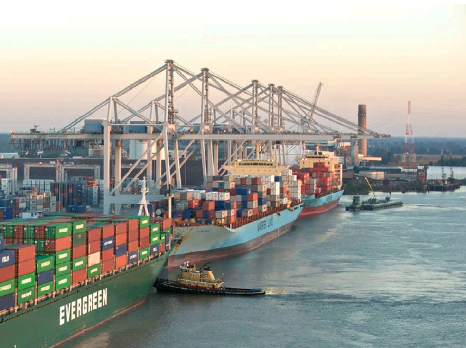
The Port of Savannah’s Garden City Terminal, which spans 1,200 acres, has the capacity to handle an increased volume of cargo from super post-Panamax vessels.
