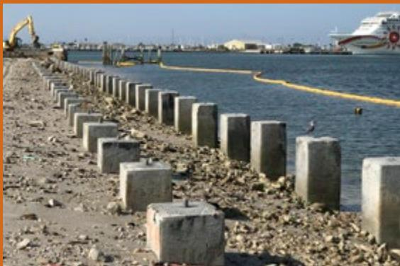
Work is underway on a multipurpose cargo berth project at Florida's **Port Canaveral** that will provide the infrastructure and capabilities to handle a wider range of heavy and oversized cargo, including commercial spacecraft components. Scheduled for completion in mid-2019, North Cargo Berth 8 on the port's north side is designed and engineered as a multimodal/intermodal berth that will provide flexible capacity and capability to accommodate more diverse commerce at the port.
