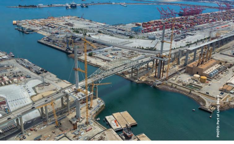
The Gerald Desmond Replacement Bridge, which is being constructed alongside the current bridge, will span the Port of Long Beach's back channel. Additional traffic lanes will expedite truck traffic to the port, and a higher clearance will accommodate new, larger cargo ships.
