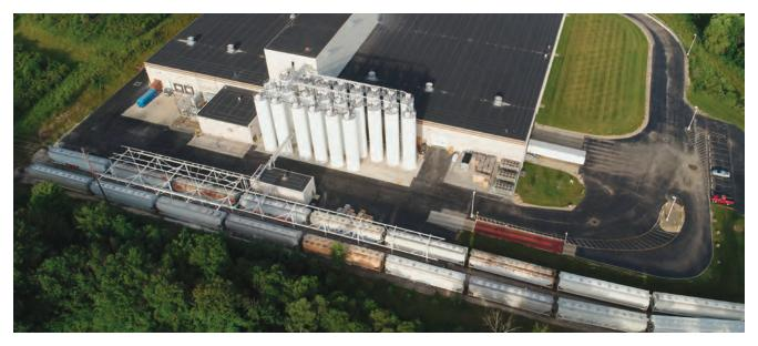
Aurora Plastics' Streetsboro, Ohio, plant, which has the capacity to hold 18 rail cars, relies on rail transportation for raw material delivery, particularly for its five most used resins.
