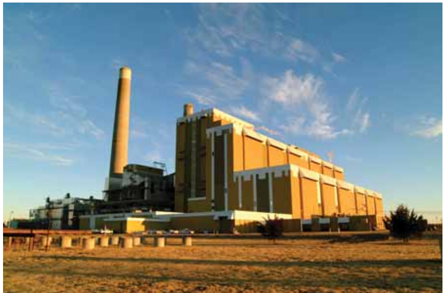
Nebraska's largest power plant, Gerald Gentleman Station, consists of two coal-fired generating units, which together have the capability to produce 1,365 megawatts of power. NPPD built a second rail spur to the plant in 1994 so coal can be shipped directly from UP or BNSF railroad lines.
